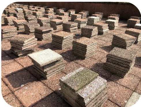
Silex tiles 4,350sqm, 540t Reuse on site
