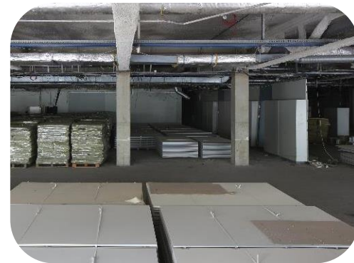
Wood panels 13,000sqm, 150t Reuse off site
