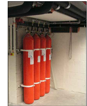
2 Blussysteem Proinert 50% Ar +50% N 2 Syst. d'extinction Proinert 50% Ar +50% N 2
