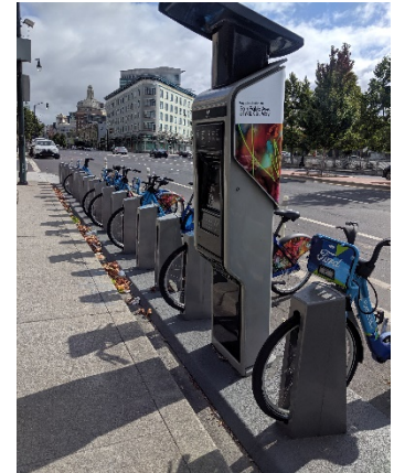
Figure 10: Gap between kiosk and sidewalk curb
