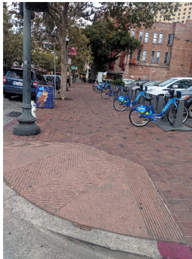
Figure 9: Diagonal curb-cut at Washington & 8th St without truncated domes
