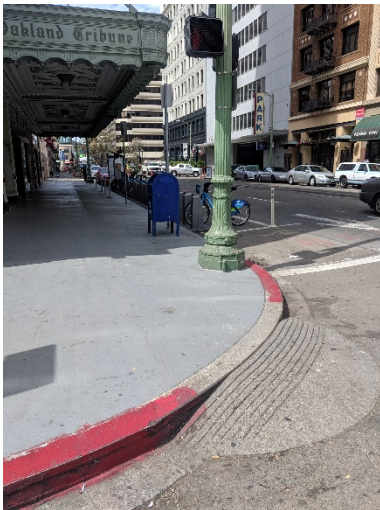
Figure 8: Built-Up Curb Ramp at Franklin & 13th St
