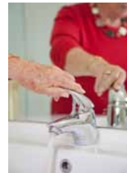
Single spout, lever taps are easy to use especially by people with arthritic hands.
