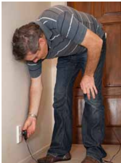
When powerpoints are this low they are difficult to reach and may lead to a back injury for less mobile or tall occupants. This powerpoint at 200mm from the floor to the centre of the powerpoint is below the required Lifemark Design Standard of 300mm and significantly lower than the preferred Lifemark Design Standard of 500 – 1200mm.
