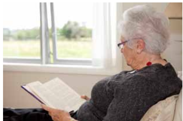
These windows meet the Lifemark Design Standard by being lower than 1200mm above the floor. The woman is able to sit up in bed reading while at the same time she can see out of the window.
