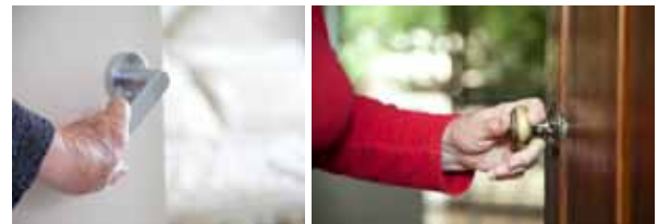
A lever handle is much easier to use than old fashioned knob handles.
