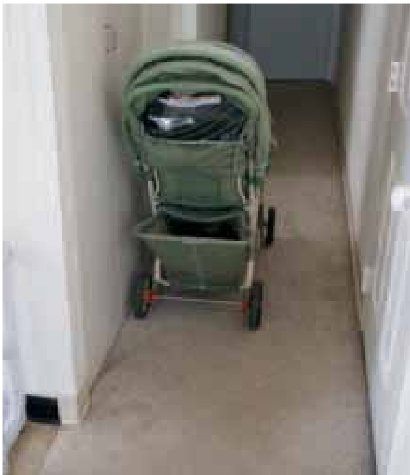
A clearly sub-standard corridor with restricted accessibility.
