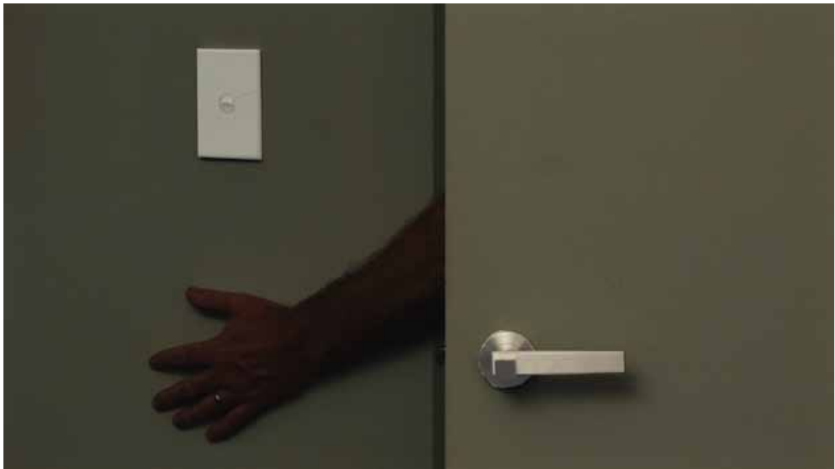
This light switch is not horizontally aligned with the door handle and results in the person feeling around to try to find it in the dark.
