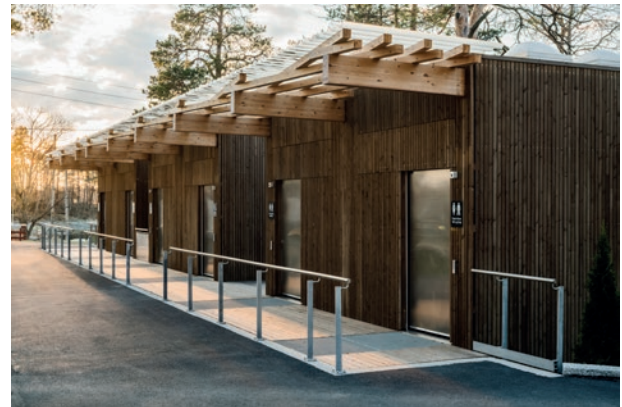
BETTER FOR ALL: "It is apparent that universal design can be used as a solution that is both inclusive and better for all," writes the jury that gave Solvik Camping the innovation award. (Photos: Damian Heinisch/Flux Architects)
