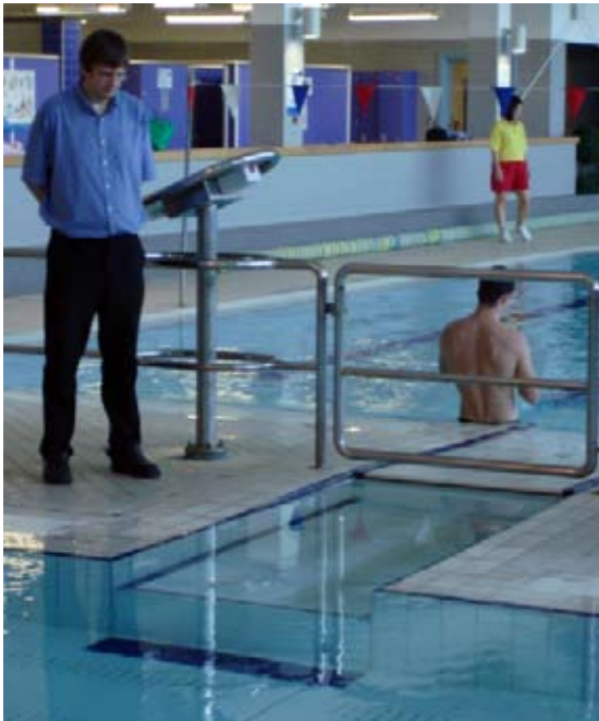
Submersible platform lift at Craven Pool, Skipton
