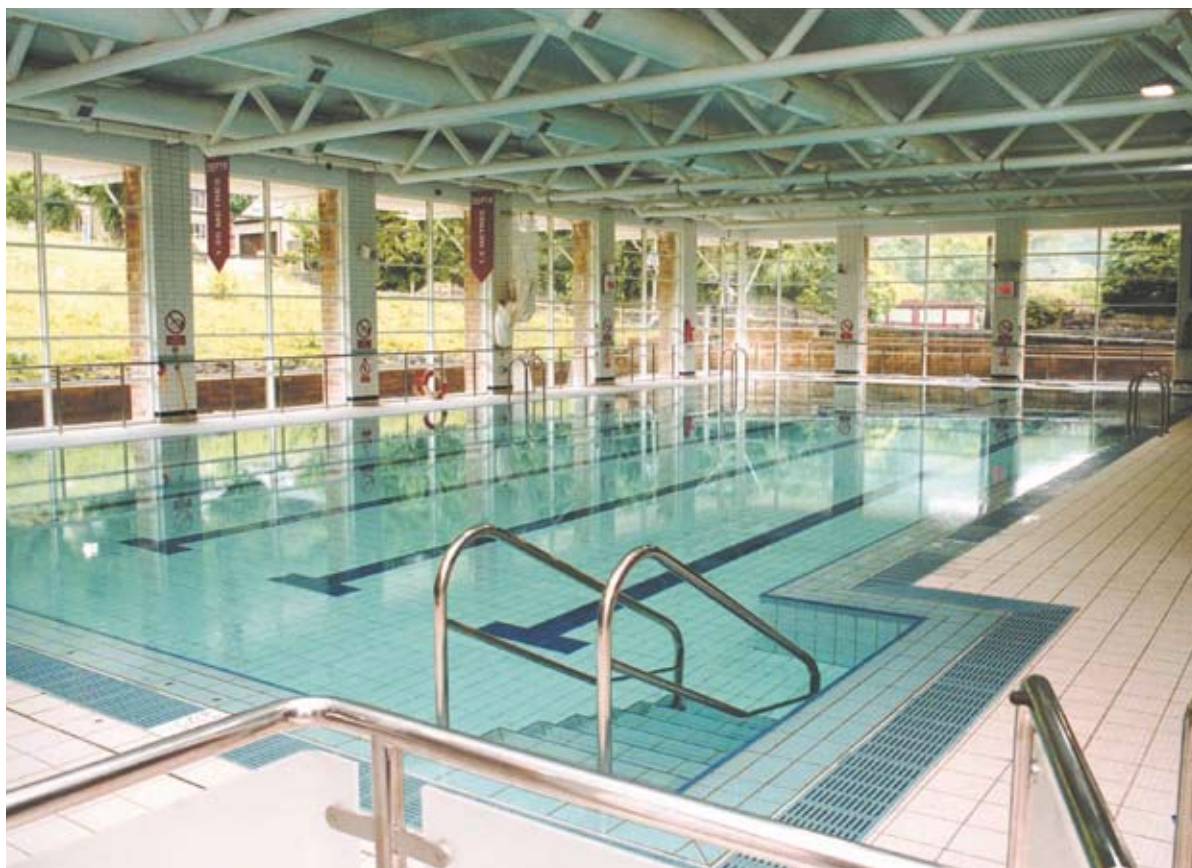
Todmorden Sports Centre – built-in steps incorporated into the pool surround
