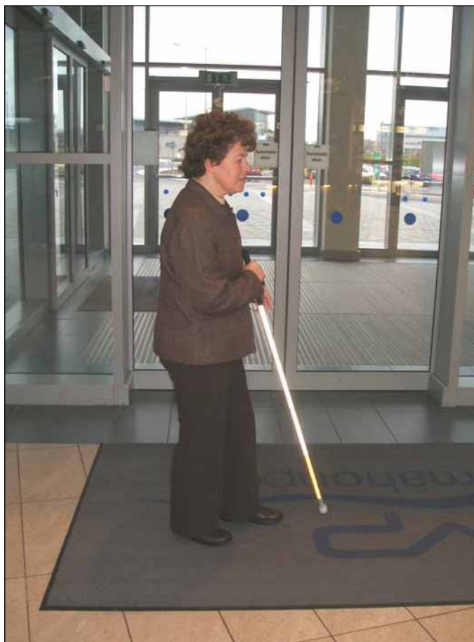
Image 4.1 Example of correct floor mat at building entrance.
