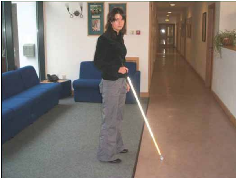
Image 4.2 Example of junction between carpet and linoleum-type flooring, which differentiates the circulation route from the seating area.
