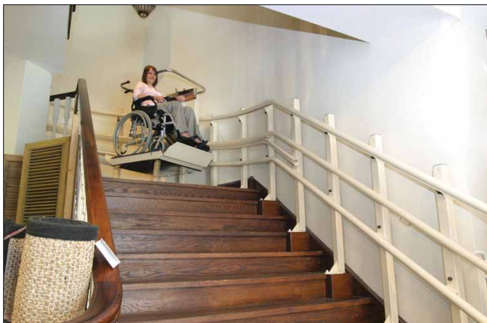
Image 3.15 Example of an inclined platform stairlift viewed from below.
