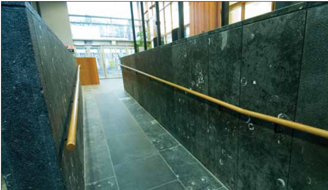
Image 3.3 Example of ramp with selected stone floor surface and contrasting wooden handrails.
