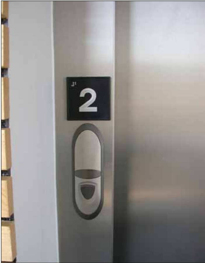
Image 3.7 Example of floor number signage fixed to elevator door frame.
