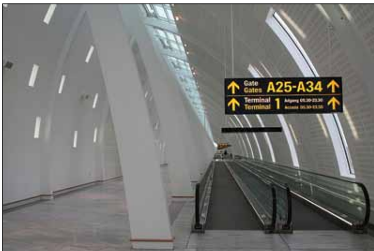
Image 3.26 Example of travelator with emergency stop button and guard rails alongside pedestrian corridor.
