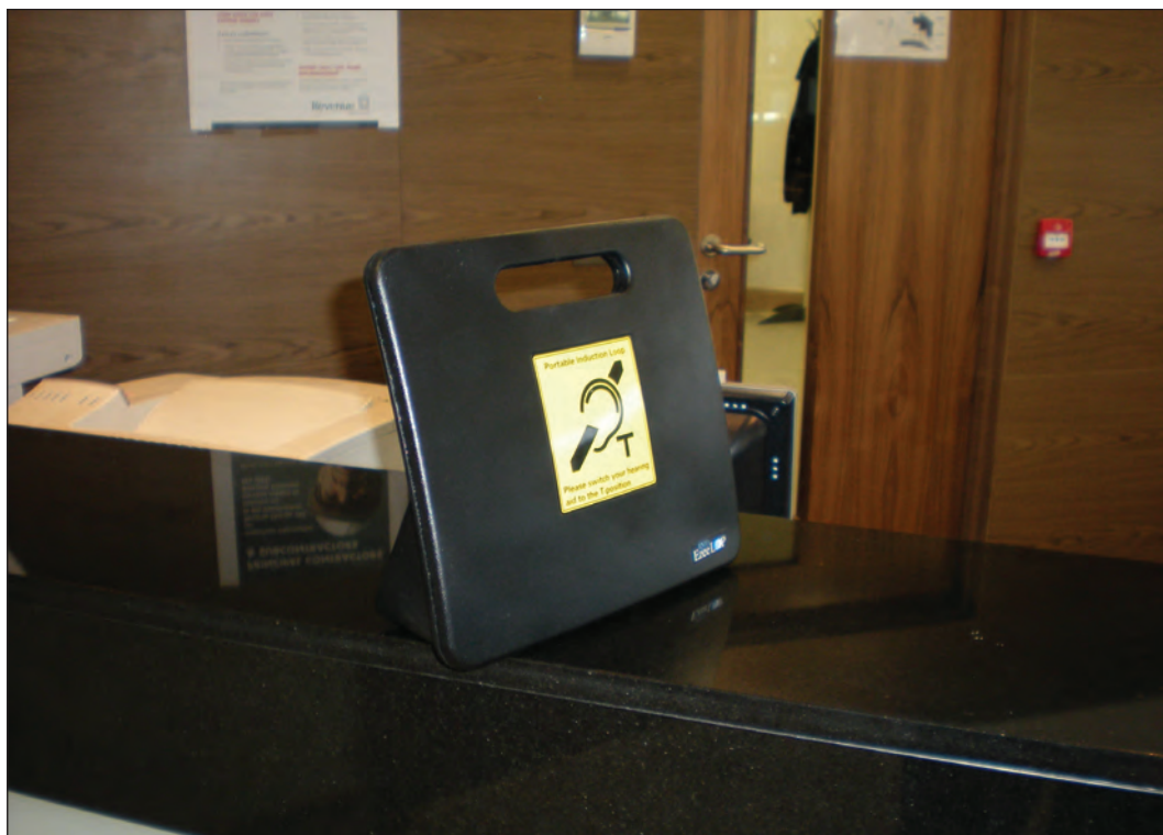
Image 2.8 Example of signage for an induction loop at a reception desk.
