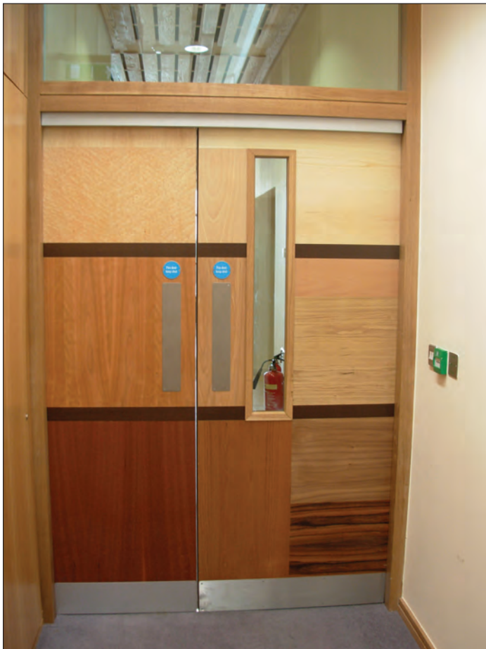
Image 2.22 Example of door with finger and kick plates.
