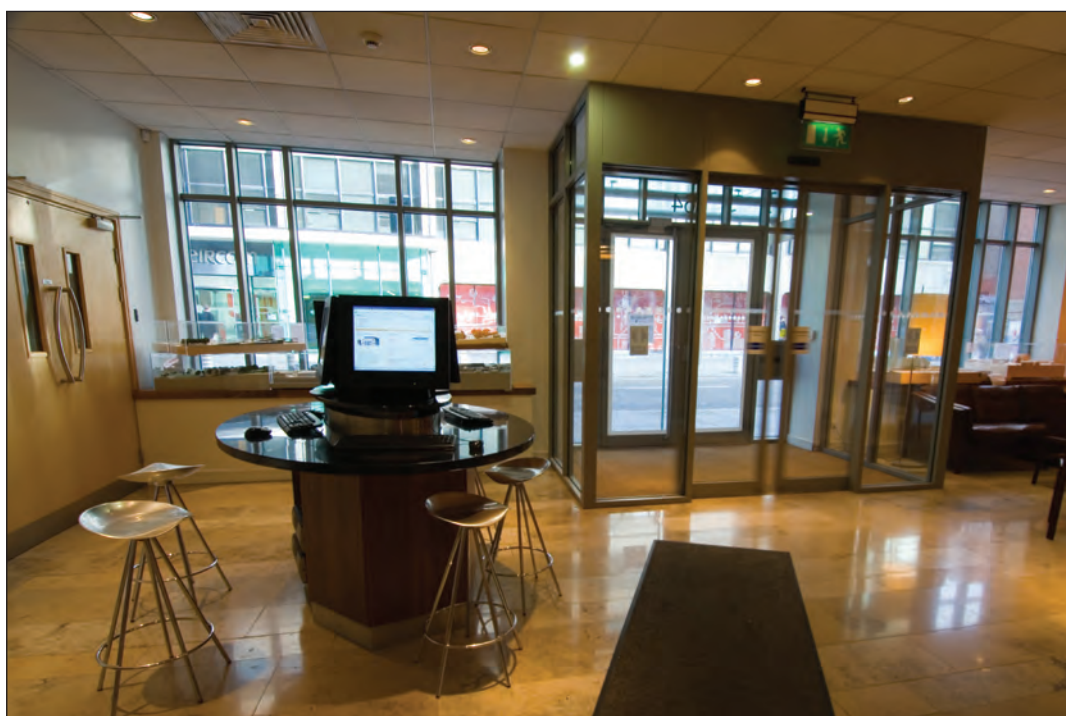
Image 2.4 Example of glazed lobby with automatic sliding doors.
