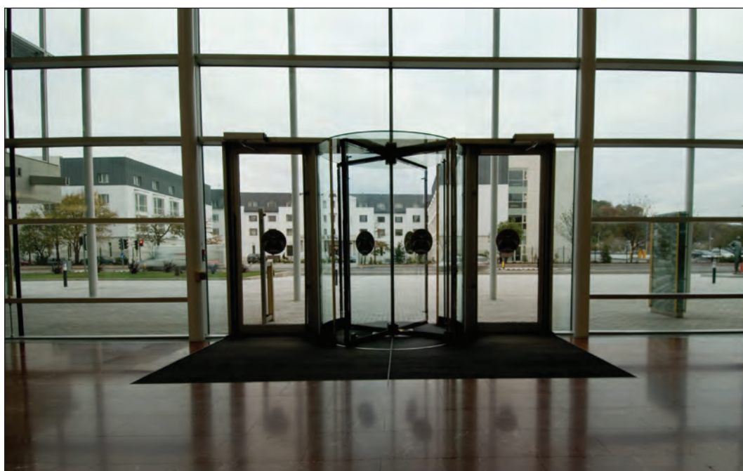
Image 2.19 Example of revolving door with a hinged automatic door located either side.
