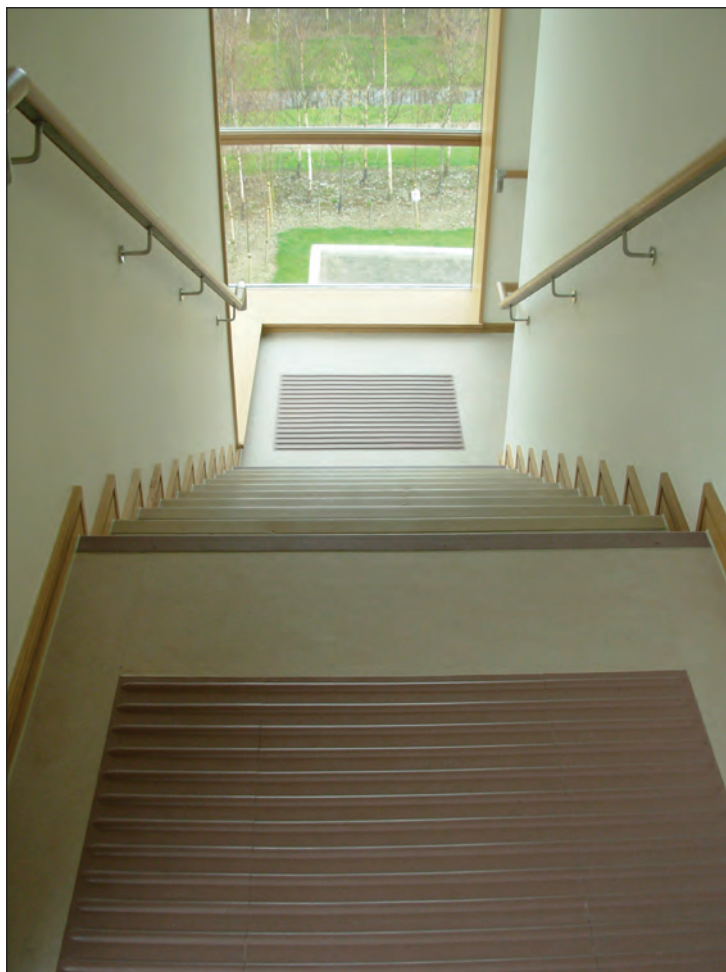
Image 2.15 Example of tactile surface at top and bottom of steps.
