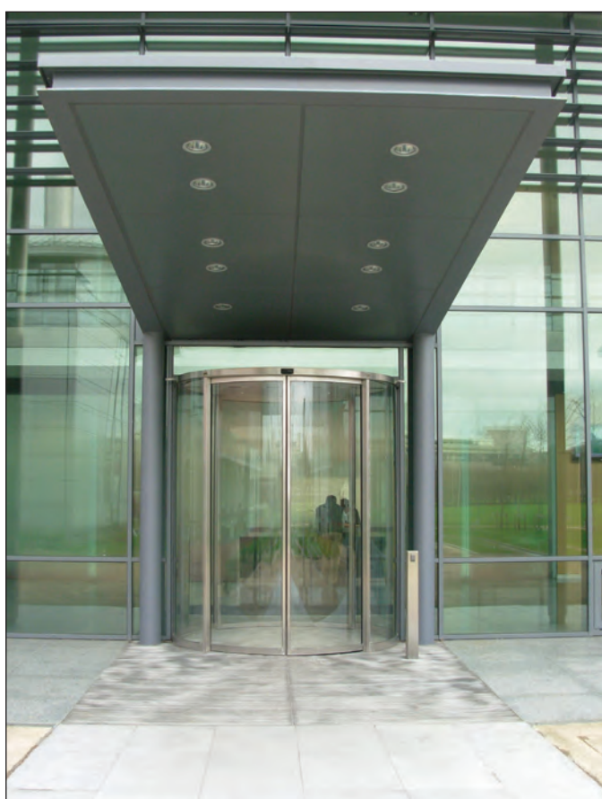
Image 2.2 Example of an entrance canopy.
