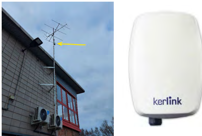
Figure 3: left: Gateway installed to an existing antenna pole – right: Installed gateway
