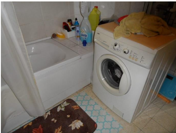
wasmachine in beschermingsvolume 2
